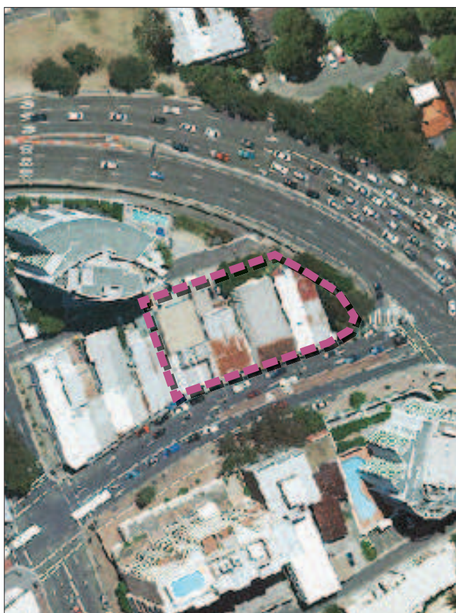
Figure 9.7 Key Site 3 - 570-578 Oxford Street
